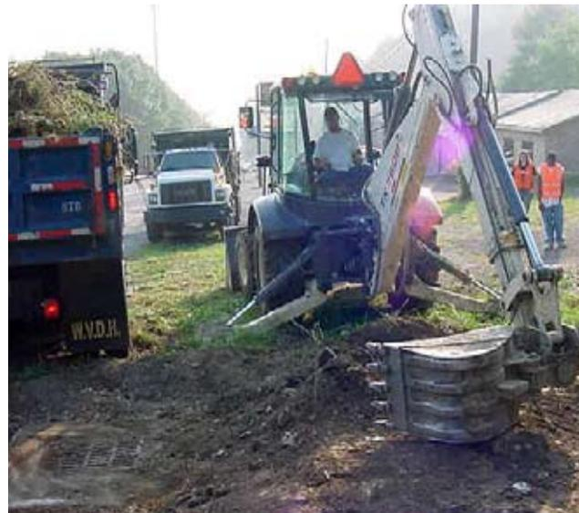
trench to the appropriate depth and width for pipe installation. With PowerTilt, they could tilt the bucket to level and make the bed for the open top drain or the drop inlet level. “With PowerTilt you can save so much time and effort by simply positioning your bucket instead of
